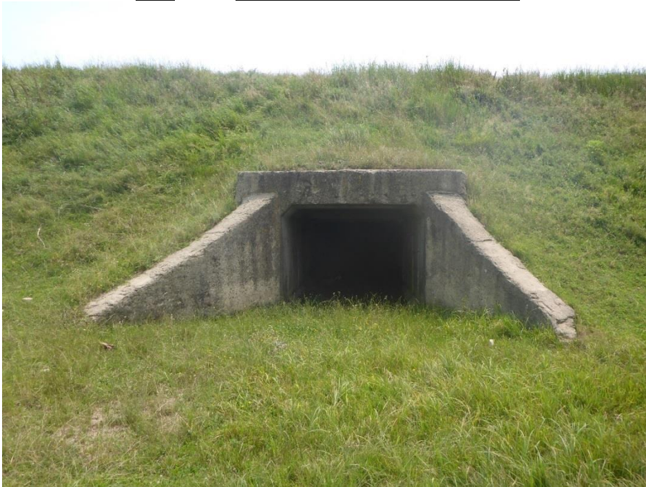
Box Culvert 2.00x2.00 km: 20+697.13
