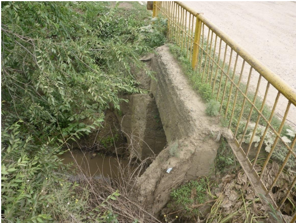
Box Culvert 2.50x2.50m km: 8+086.81
