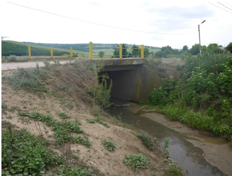
Box Culvert 3.00x2.00m km: 8+621.03
