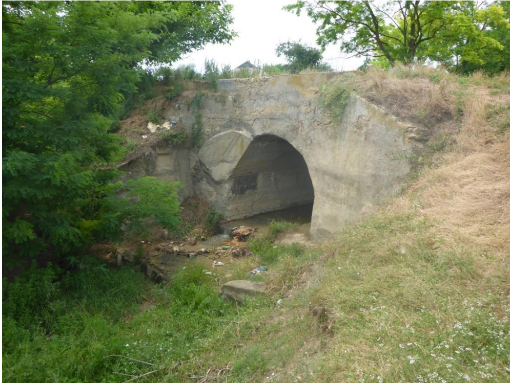
Box Culvert 1.50x2.50m km: 6+288.77
