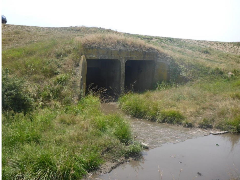
Box Culvert 2x1.50x1.50m km: 16+469.22
