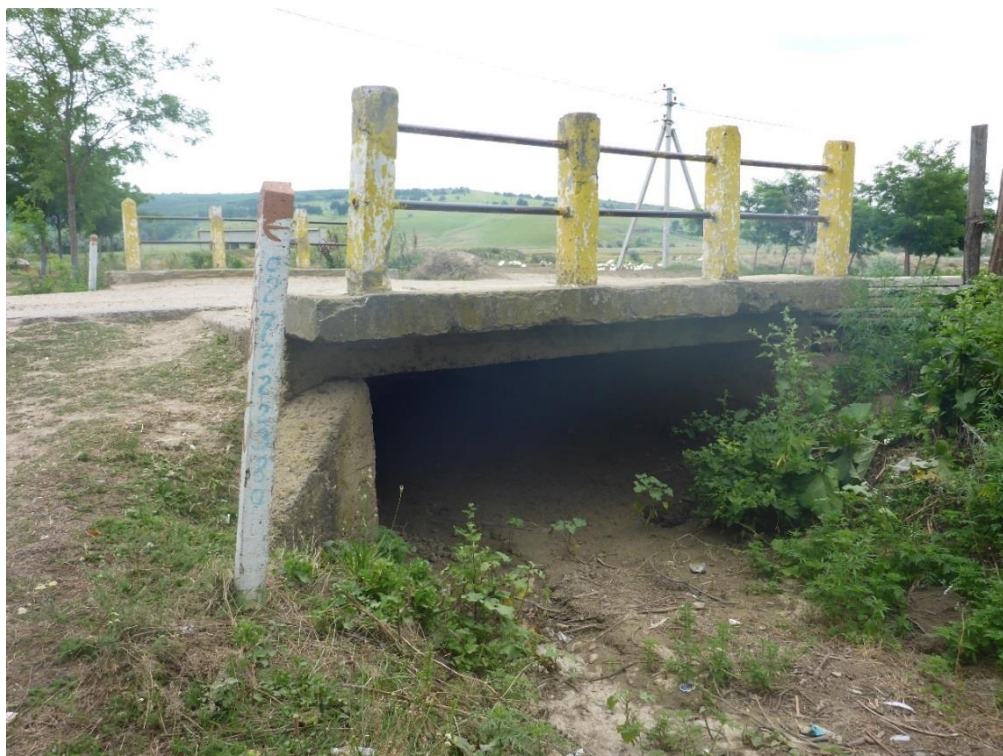
Box Culvert 3.00x2.00m km: 8+621.03
