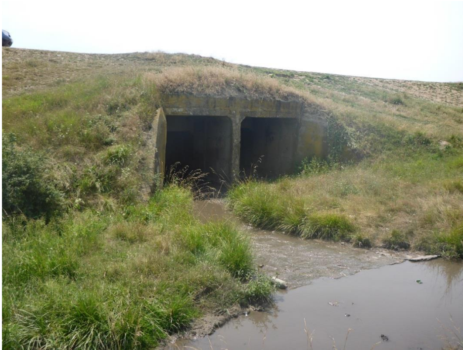
Podet casetat 2x1.50x1.50m ch: 16+469.22
