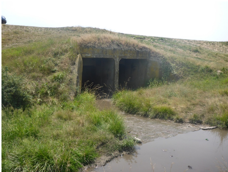
Podet casetat 2x1.50x1.50m ch: 16+469.22
