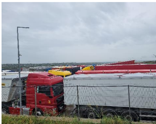
Custom service control platform. Full parking area
