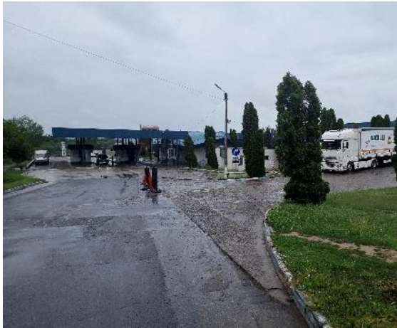
Car/passenger entrance area
