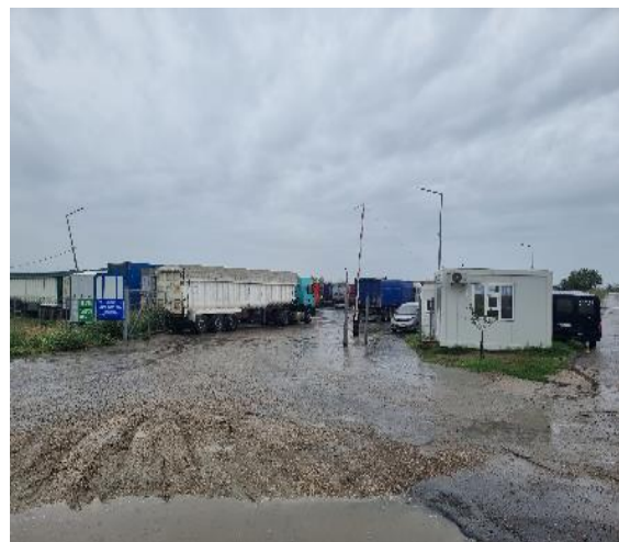
Custom service control platform entrance
