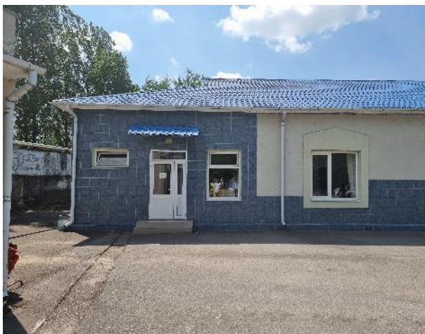
Former Center for training. Actually, unused as training center is in Chisinau
