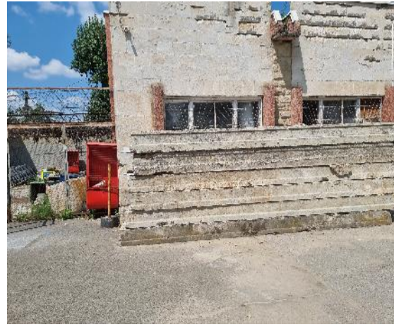
Old building, unused
