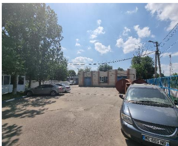
Parking area and old building (storage area)
