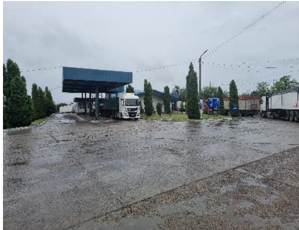
Cargo/trucks entrance area
