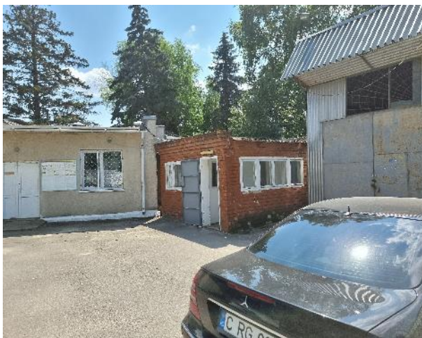
Old building, unused
