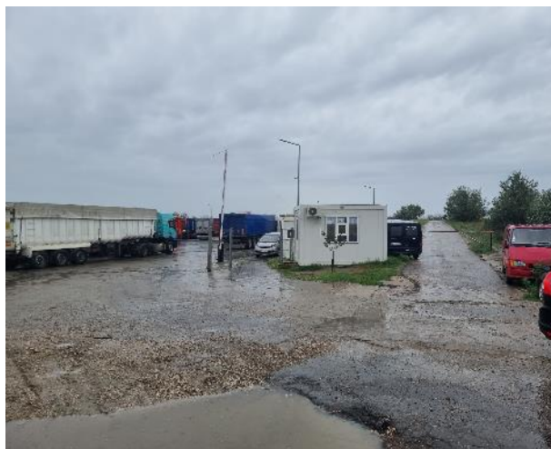
Custom service control platform entrance
