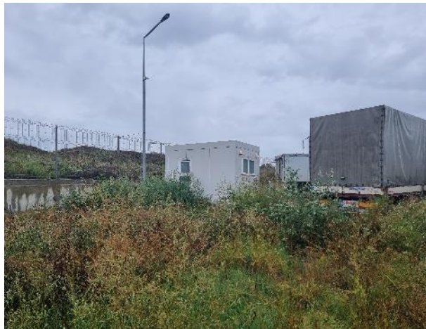
Sanitary facility – not working.
