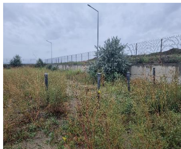
The area of platform needed to be covered by concrete – wastewater pit
