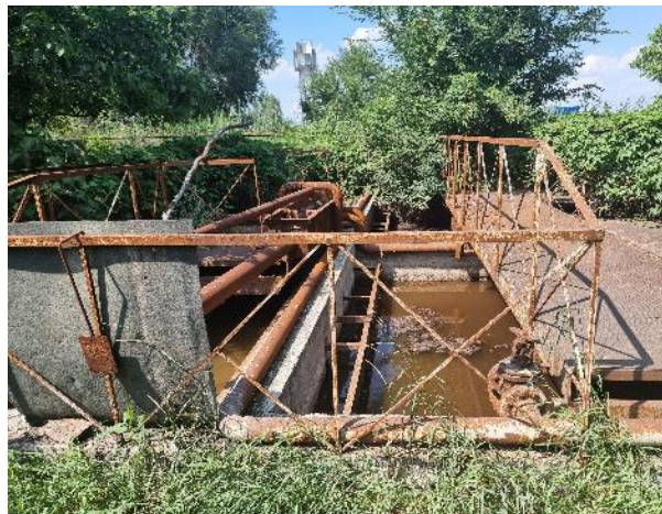
Primary treatment basins, equalization tanks
